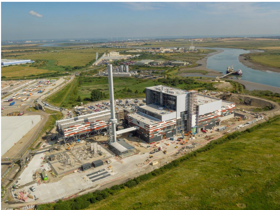
Figure 6.1 – K3 construction progress at July 2019.
